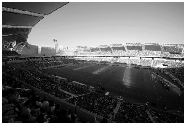
Dunas have depth in themselves and that depth is used to generate a support structure from *within* the roof section itself. It doesn't need any external support from above or below. The petals are apparently made of steel trusses, coated with aluminium tiles on the outside and with a PVC pre-stressed membrane in the inside. But however the structure works it strikes me as an absolute revelation in stadium design. If you are interested in reading a bit more about it – see below.
